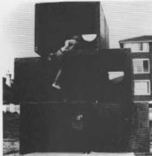
This cliff-dwellers' unit was designed by Professor Peter Spooner of the Architecture Faculty, University of New South Wales, Australia. The pre-fab sewer junction boxes were assembled by the Brisbane Public Works Department.
